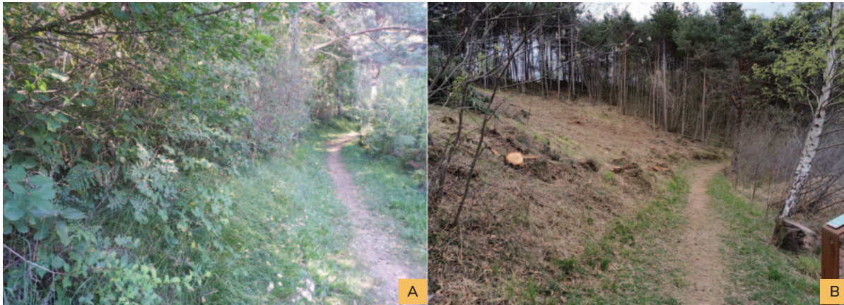
Figure 2. Site preparation at the Le Grave project site (Trento, Italy) prior to the translocation of Gladiolus palustris . A) Original state, with dense tree and shrub vegetation, summer 2023; B) Result of the clearing work, spring 2024.
