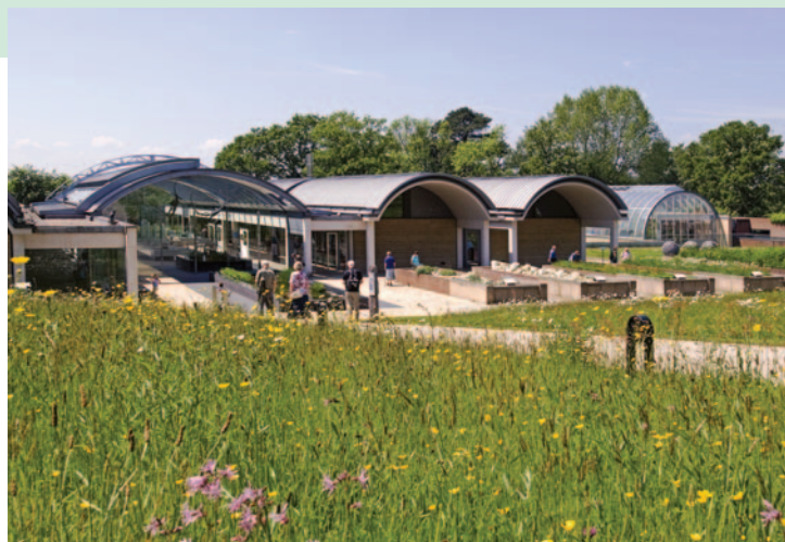
This building houses Kew's Millennium Seed Bank at Wakehurst, United Kingdom. © RBG Kew.
