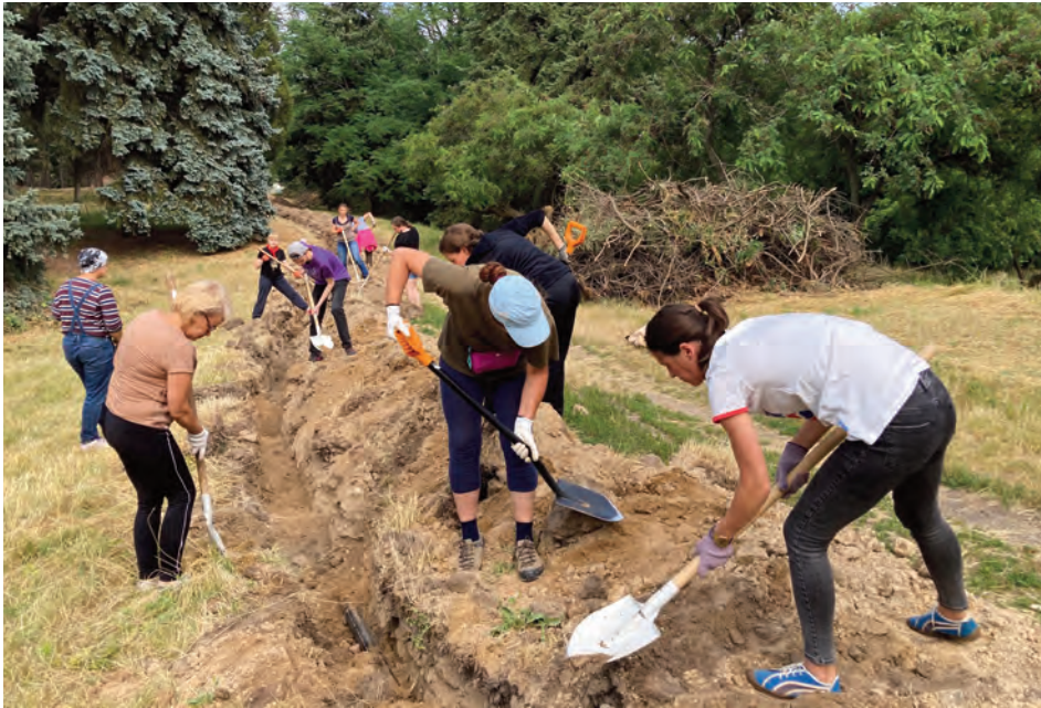
Volunteers helping to build the irrigation system (Valentyna Sliusar)
