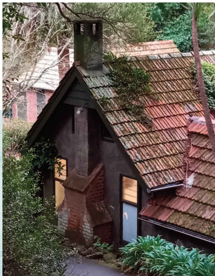
Cracked chimney of the gardeners' depot and separating from the building at Wellington Botanic Garden, following the Kaikōura earthquake in 2016. (David Sole)
