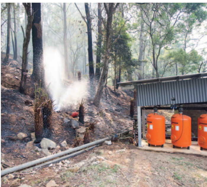
Water leak of the main Garden supply line following bushfire at Mount Tomah, New South Wales. (Greg Bourke)
