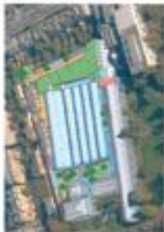
Above: Aerial view view of the proposed North West Corner redevelopment. (South Ayr District Council)
