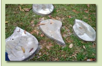
The walkway is comprised of leaf shaped stepping stones made from cement. This provides a raised area for people to walk on when the ground below is very wet (in the rainy season). Leaf and flower imprints have been cast on the top layer of cement.
