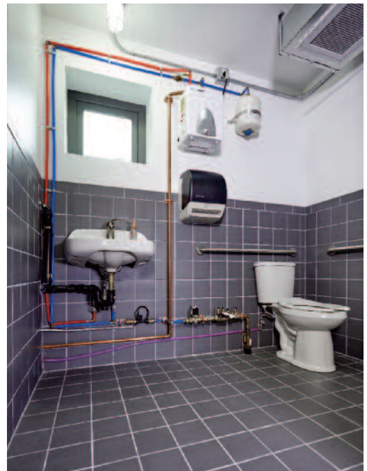
↑ Exposed water pipes within the SEED Classroom that are used as educational aids for the teaching of water security ©Banko Media, Inc.
