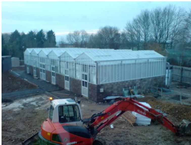
Fig 1 New glasshouses under construction
