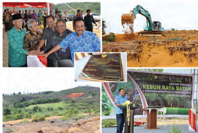
Ground Breaking Batam Botanic Gardens on August 28, 2014 by the Minister of Public Works of Indonesia Ir. Djoko Kirmanto, Dipl. HE.
