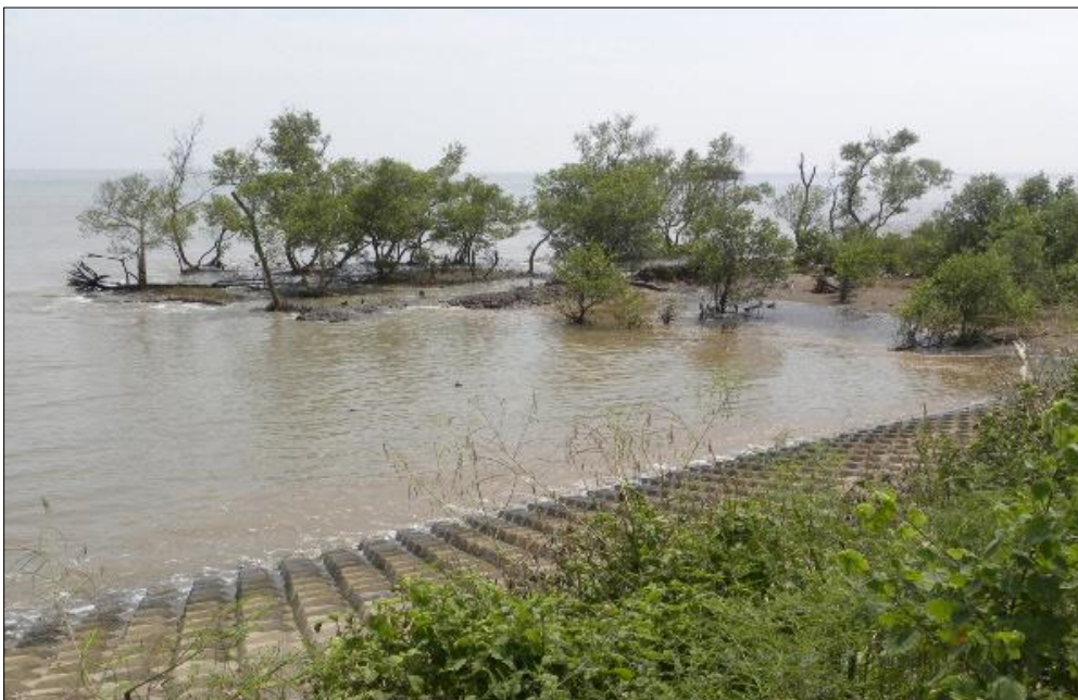
Figure 1. Coastal area in Vietnam with revetment on clay soil and remnant pocket of mangrove
