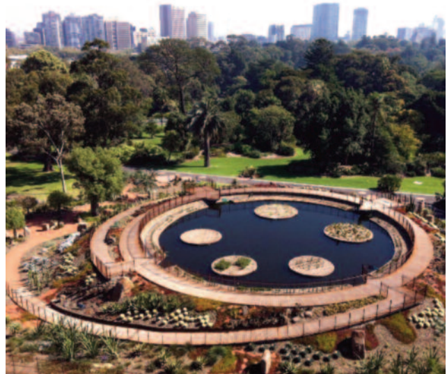
Guilfoyle's Volcano Project, Royal Botanic Gardens Victoria (RBGV), Australia – a model of project management – constructed from the renovation of a century-old reservoir and integral part of RBGV's water recycling plan. (Image: Katie O'Brien)
