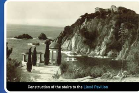
Construction of the stairs to the Linna Pavilion
