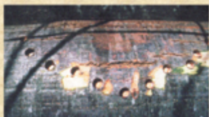
Pellets are placed into drilled holes around lesion
