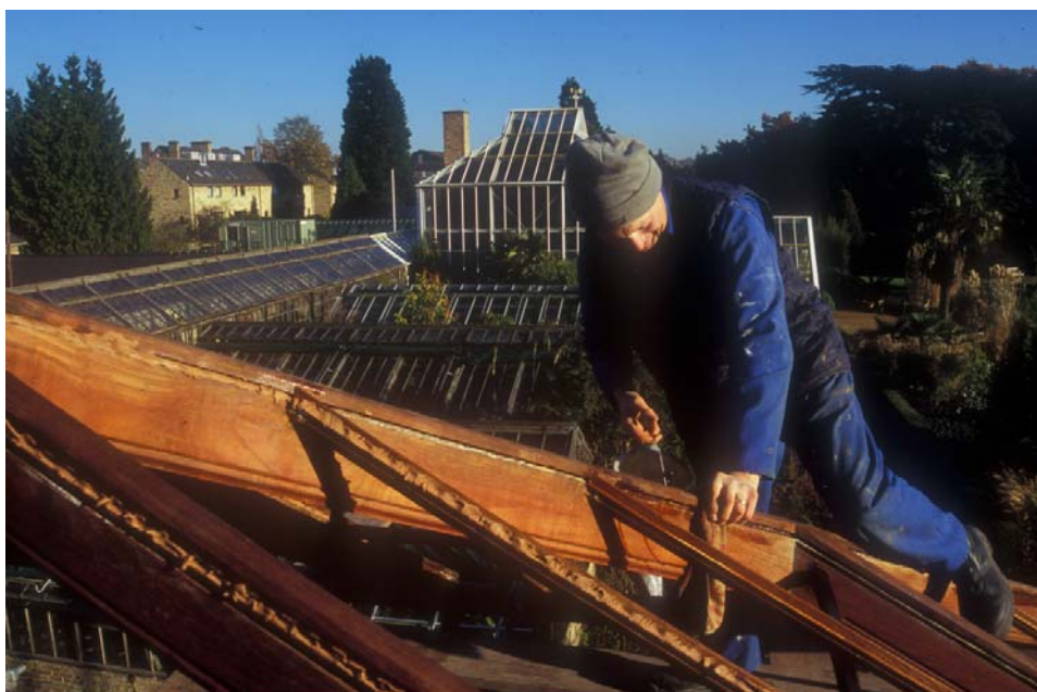
Figure 2. - The original timbers of the Temperate House roof restored to their former glory pictured during reglazing. The corridor leading to the Palm House, rebuilt in steel and opened in 1989, is shown beyond.
