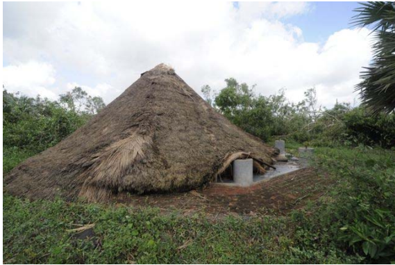
Education Pavilion Roof Blown off
