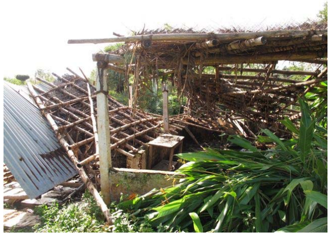
Parking shed destroyed
