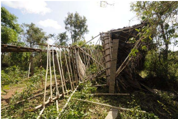
Watchtower Blown Down
