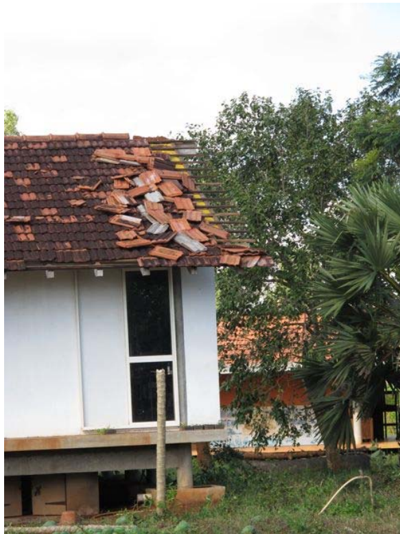
The Seed Room Roof damaged
