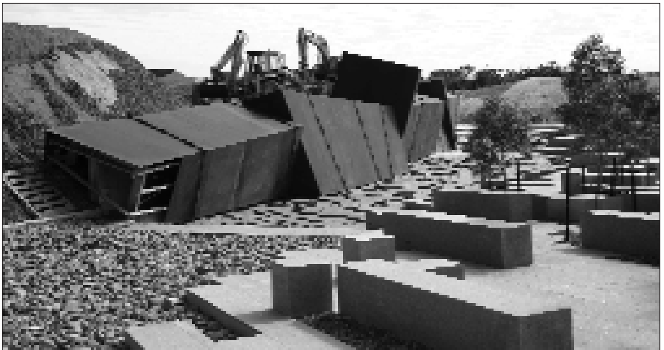
Right: Escarpment wall sculpture within the newly constructed rockpool waterway
