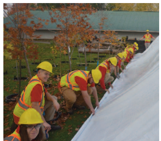
↑ Second-year students installing winter poly on the cold frames in the retail nursery ©Michael Pascoe
